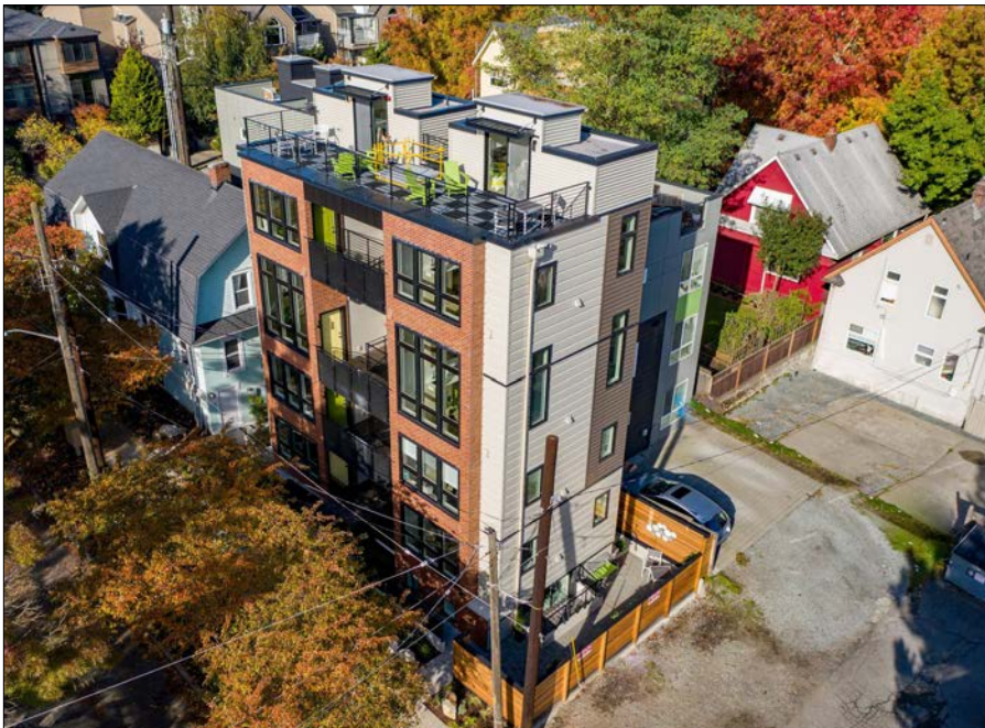
A multifamily building in Seattle with a single staircase, which allows for construction on smaller parcels and more diverse unit configurations serving a broader range of needs. Photo source: Sean Jursnick/X.
